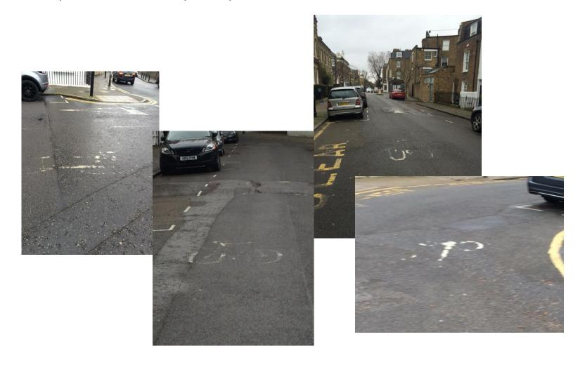
Motor vehicles move to centre of road to straddle the speed bumps: on both the two way and one way / cycle contraflow sections
